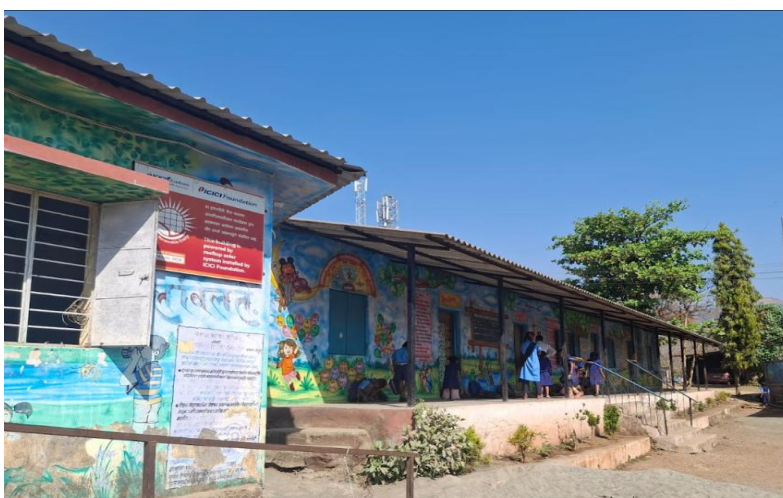
Figure 20 A school in Maharashtra impacted by the solar panels
